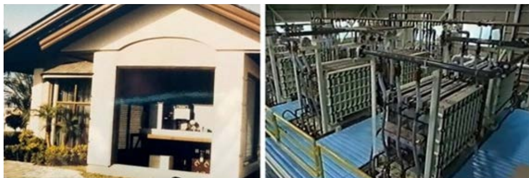
Fig 2: Early VFB Field Trials: (Left) VFB installation in Demonstration Solar House in Bangkok in mid-1990s; (Right) 200 kW/800 kWh VFB at Kashima-Kita Electric Power Station in Japan in 1996–97. Photos courtesy Rui Hong (left) and Chris Menictas (right).
