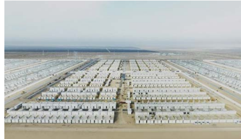
Fig 6: 200 MW/1000 MWh VFB in Xinjiang, China. Published with permission from Xingchen New Energy.
